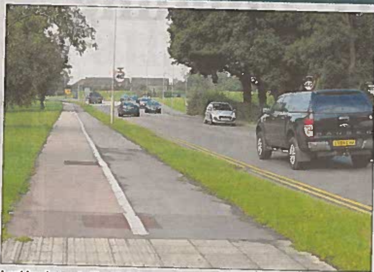
Looking towards the Matalan roundabout from the Hilton Road junction
